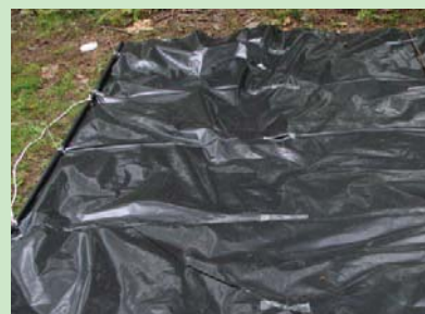
Construction of a 6-mil polyethylene benthic barrier.
